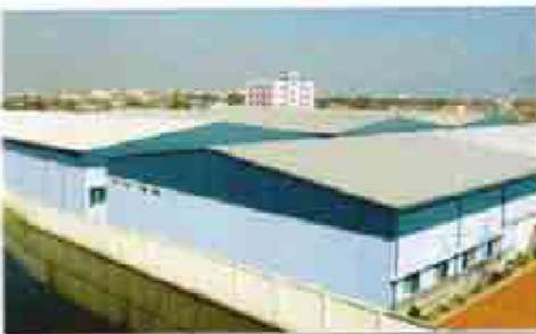
Power Swaters Ltd. 1,64,591 Sq. (Waste Factory) Kalyandurg
