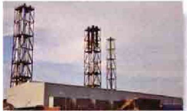
Energypac Power Generation Ltd, 44,945 Sft / Faridpur
