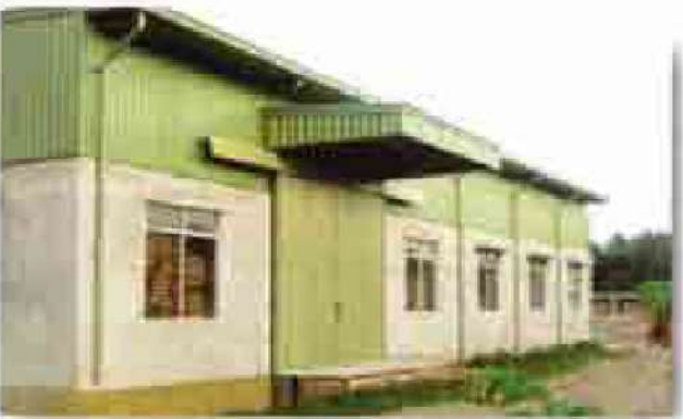
Fakhruddin Textile Mills Ltd. 4,212 Sft. (Generator Building) Sreepur, Sreepur
