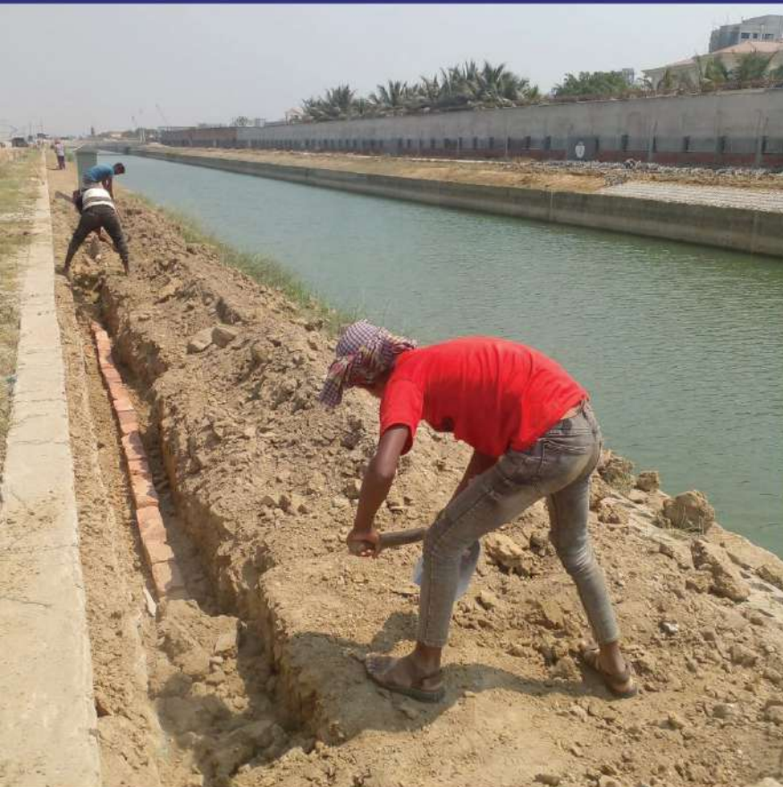
Electric Cable laying at 300 feet, Purbachal
