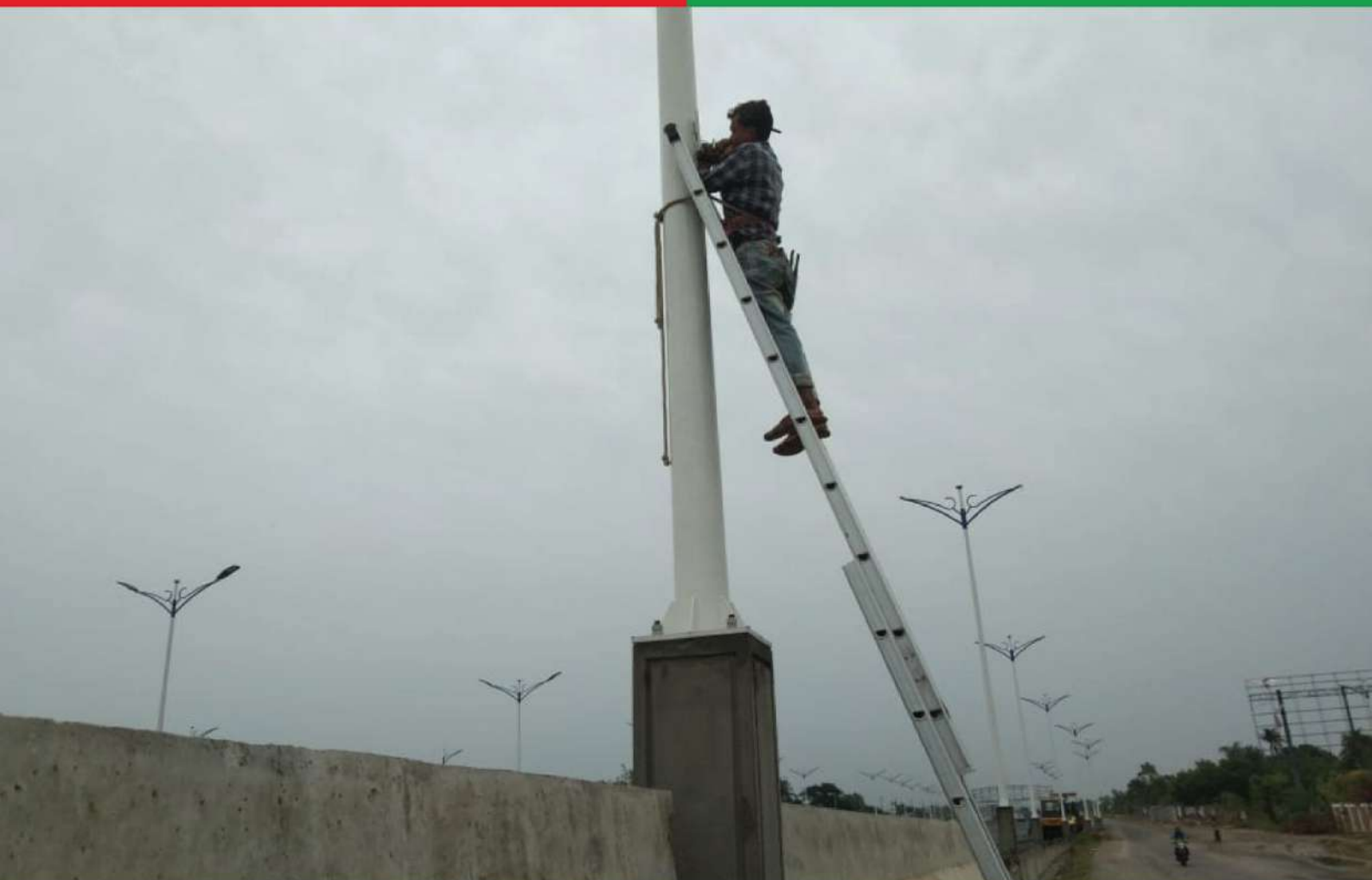
Electric Cable laying at 300 feet, Purbachal
